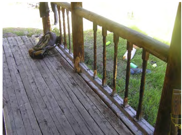
Figure 27: The guardrails are set between the log columns of the east porch.
