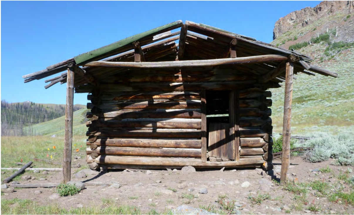
Figure 13: The cabin as seen from the east.
