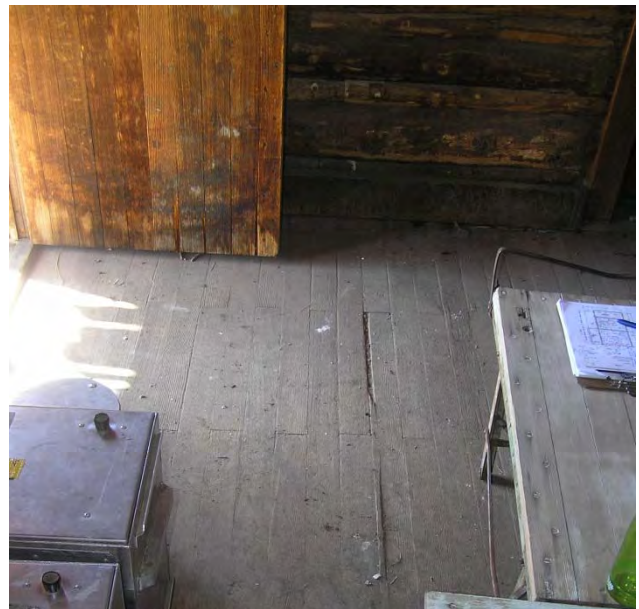
Figure 53: The Living Area flooring is splintered near the entry.
