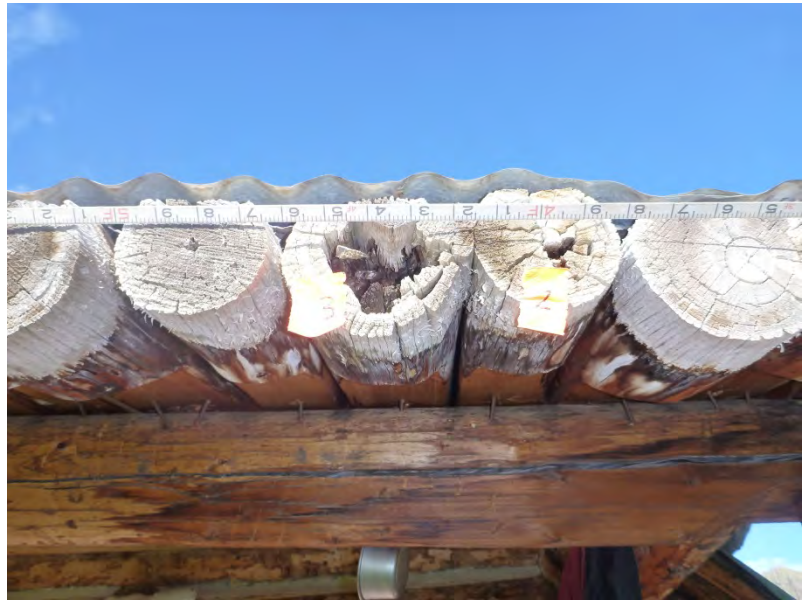
Figure 7: Deteriorated log rafter tail (pole) ends at the east porch.
