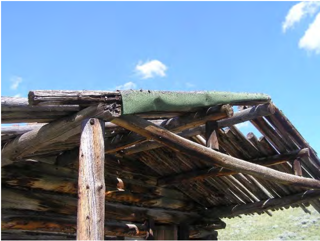
Figure 62: The roofing was pulled over the rake logs, as depicted on this south log of the entry porch.
