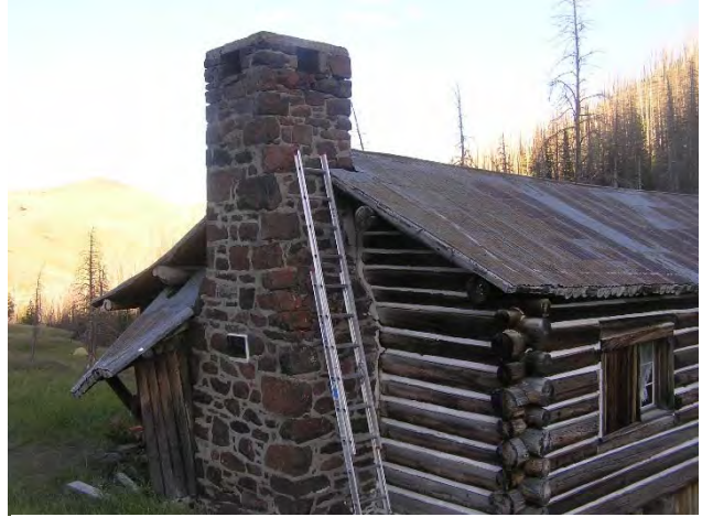
Figure 18: The stone chimney anchors down the north end of the Lodge. Photograph taken looking southeast.
