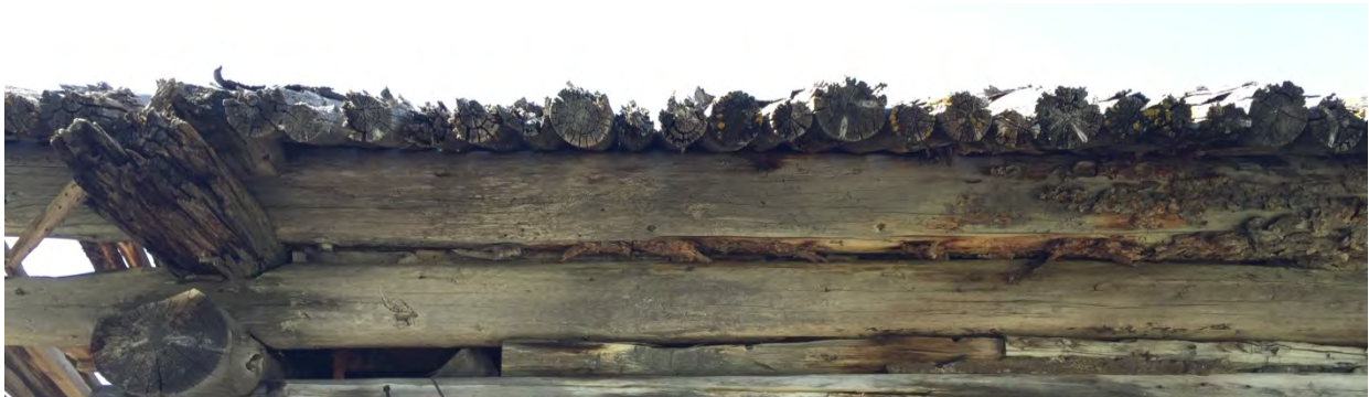
Figure 15: Roof poles at the overhangs are severely deteriorated.
