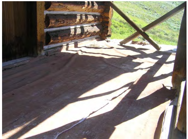
Figure 30: Painted canvas covers the puncheon flooring of the main level South Porch. It is stretched and torn.
