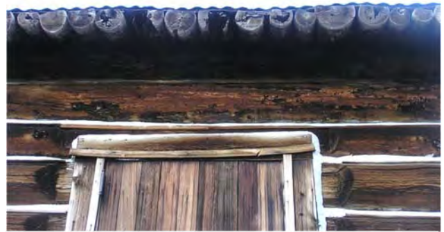
Figure 22: Daubing missing indicating natural aging & movement.
