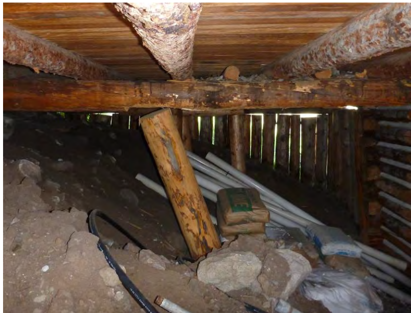
Figure 8: Displaced log column in crawl space below the living room floor framing. Erosion in the crawl space has dislodged the column base from the footing element.
