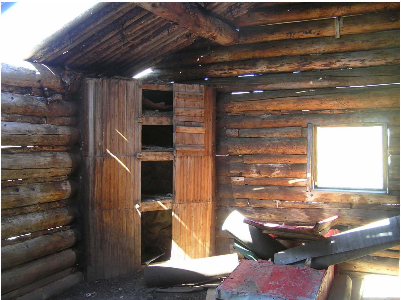
Figure 75: The Cabin interior was fitted with a wardrobe, for protective storage, in the southwest corner.
