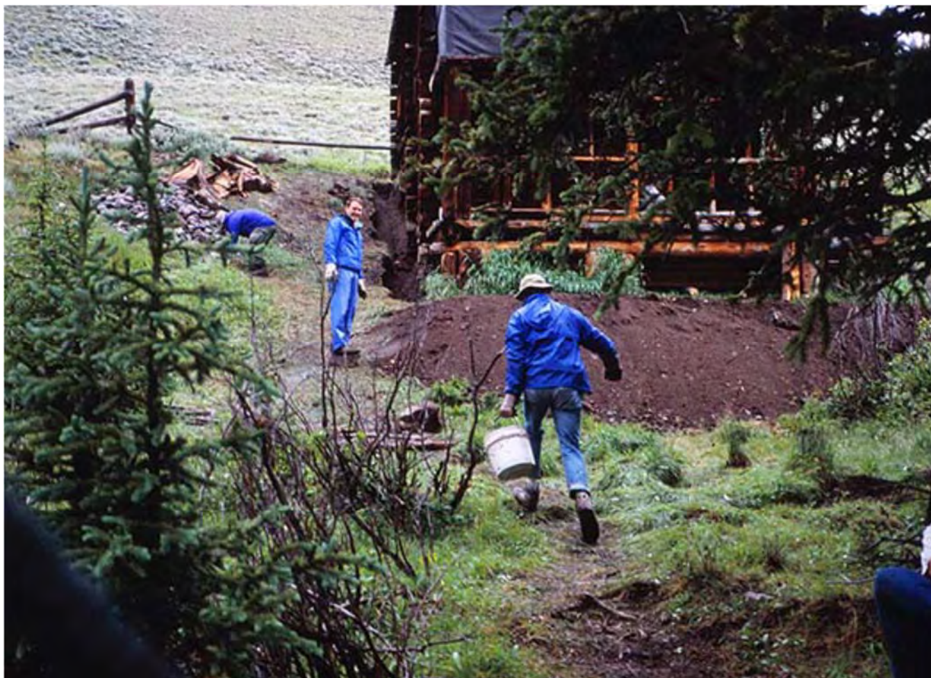
Figure 4: c.1993 shaping of drainage improvements along the west side of Anderson Lodge, with cobbles on slope ready to be put in before backfilling with sediment stock piled to the south. Workers shown carrying bucket of gravel/cobbles from Vick Creek channel for fill. Image courtesy of Mary Jane Luther, USFS retired, Meeteetse, WY.
