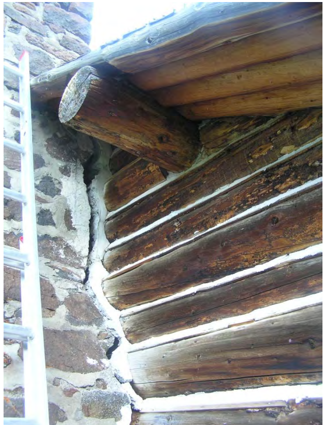
Figure 19: The building movement has caused the vertical joint between the plumb chimney and the log wall to increase over time, to as much as 2½" at the top. Note the 1993-1994 daubing mortar that filled the joint at the time.
