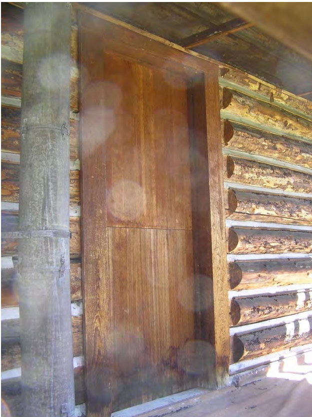
Figure 35: The entry door to the Kitchen Area from lower level porch is representative of the typical Dutch door used at the exterior of the Lodge.
