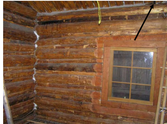
Figure 42: Dislodged vertical daubing at the southwest corner of the Sleeping Area. See also missing daubing at top of wall, designated by the arrow tip.
