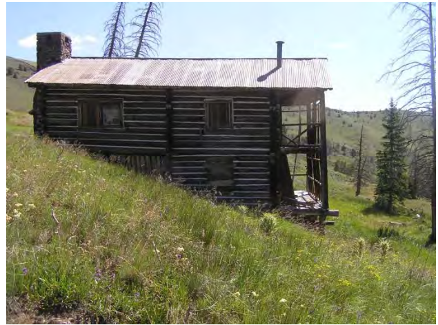
Figure 8: West elevation of the Lodge.
