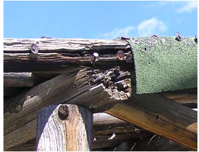
Figure 65: The rake logs and porch beams are rotted from moisture penetration.
