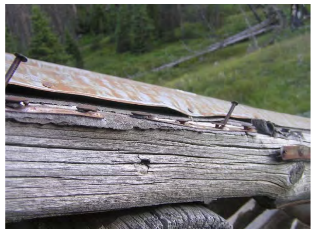
Figure 13: The roofing felt was fastened to the rake poles with metal strips that remain.
