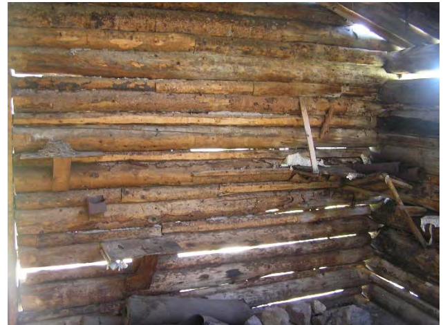
Figure 6: Erosion of daubing mortar has resulted in gaps between the Cabin's wall logs; photograph taken looking southeast.
