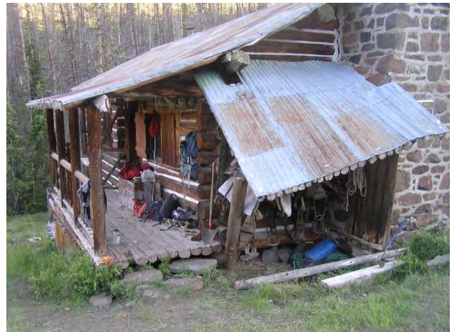
Figure 26: The east porch, as seen from the north, provides direct access to the main level Living Area.
