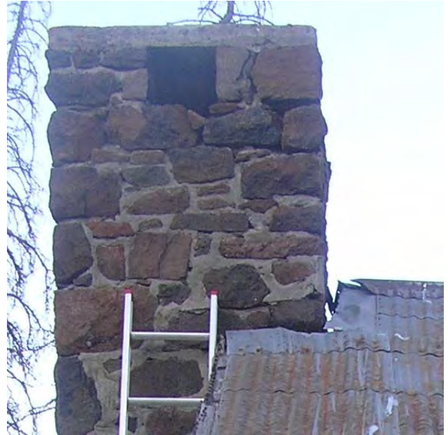
Figure 14: The building's movement away from the chimney has caused the erstwhile sheet metal flashing to fail to cover the gaps between the roofing and the chimney.
