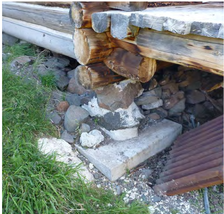
Figure 6: This rubble stone pier is located at the southwest corner of the kitchen and is supported by a concrete pad constructed during the 1991 repairs.
