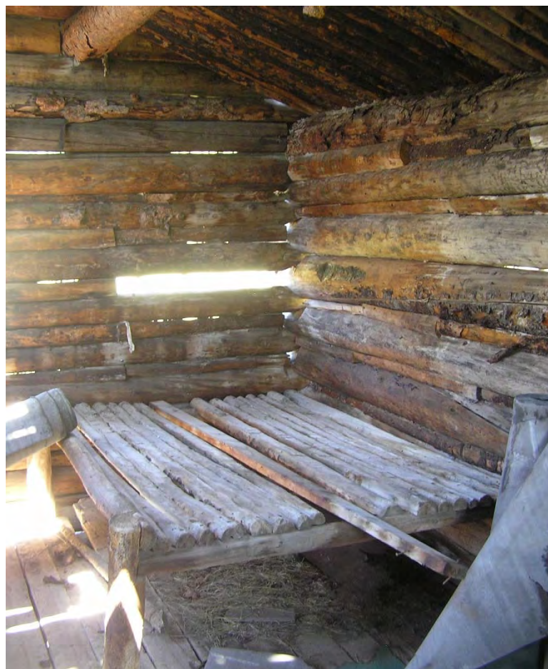
Figure 77: A rough wood log cot is built into the northwest corner of the Cabin.
