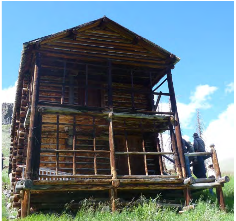
Figure 5: The South elevation of the lodge consists of the two-story porch. Photograph taken looking northeast.
