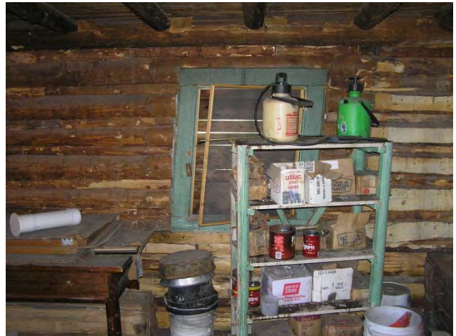
Figure 49: The window opening at the west wall of the Kitchen Area is substantially racked. The daubing that sealed the window joints has failed and fallen, due to building settlement.
