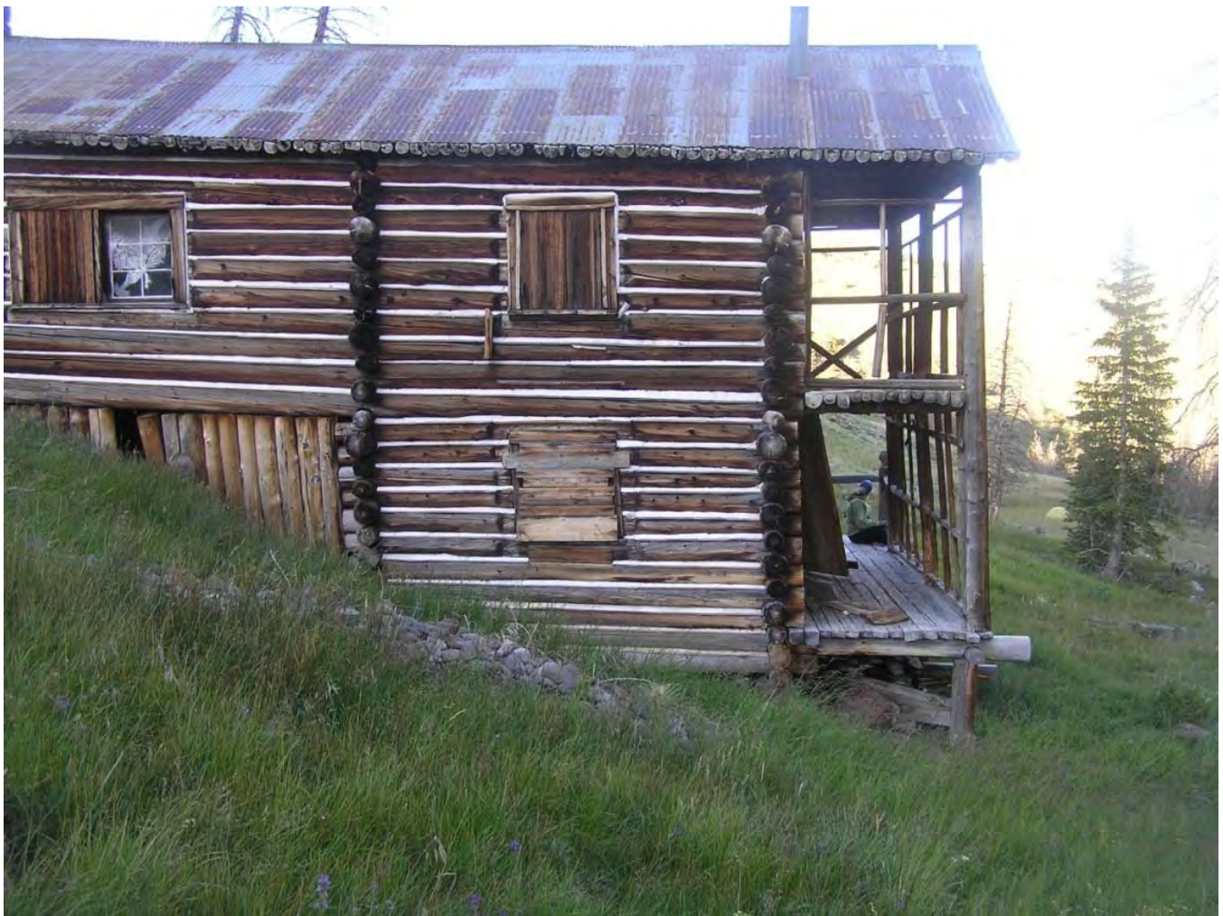
Figure 33: The windows are located on the west (as shown above) and east elevations of the Lodge.
