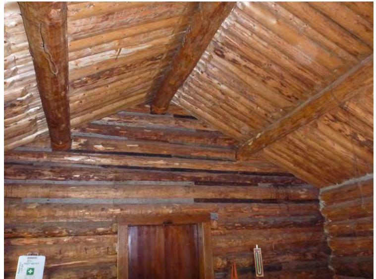
Figure 2: Roof framing seen from the living room looking south.
