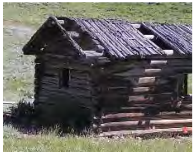
Figure 71: The west window opening is visible at the left side of this photograph.
