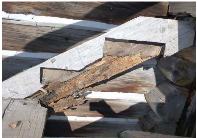
Figure 10: Failed connection of the tread logs to the stringer due to rot.
