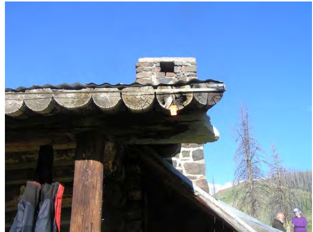
Figure 15: Deteriorated ends of roofing poles at the east porch.
