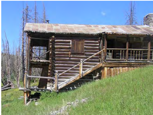
Figure 5: Anderson Lodge continues to settle to the south, as seen at the left in this photograph from the east.
