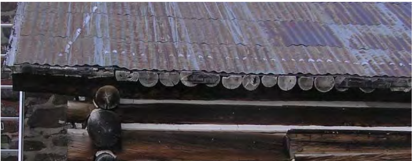
Figure 16: The roofing felt was fastened to the pole ends with a nailing strap. Much of the felt has rotten and fallen away.
