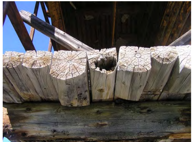
Figure 29: Rotted end of floorboard on the east end of the main level South Porch.
