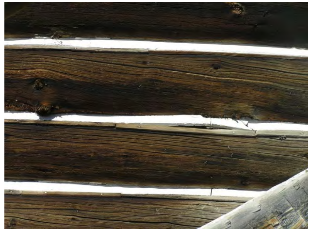
Figure 21: The daubing mortar, aided by wood daubing strips, is sloped to drain away from the log wall.
