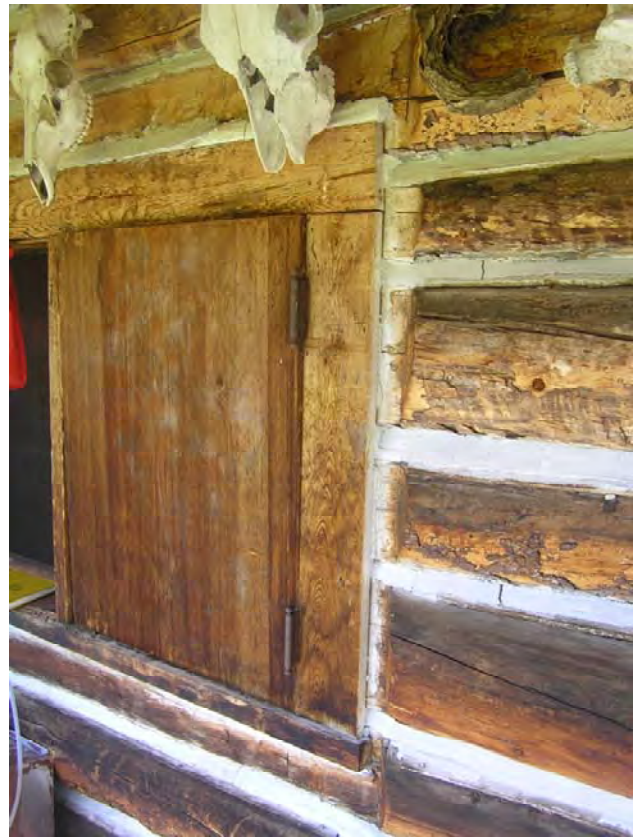
Figure 34: The typical exterior window trim is visible at the east Living Area window north of the main entry door. The typical daubing treatment around the windows (acting as a sealant to air penetration) has failed.
