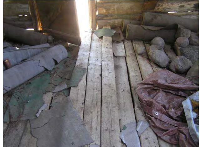
Figure 78: Looking east towards the floor boards that have popped up near the entry.
