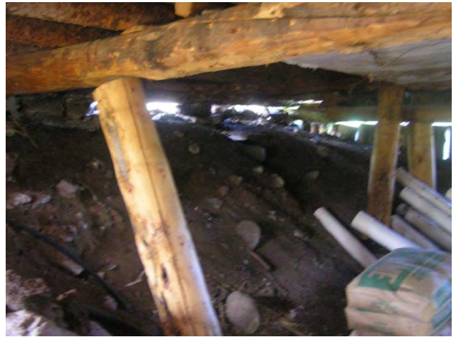
Figure 40: Plaster ceiling in crawlspace Storage Area.
