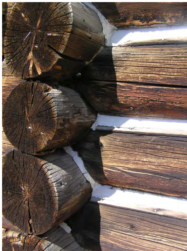
Figure 24: Building settlement has caused the daubing mortar to fail at the vertical joints of the log walls.
