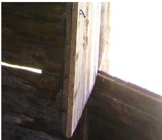
Figure 74: This interior view of the Cabin's entry door shows its construction.
