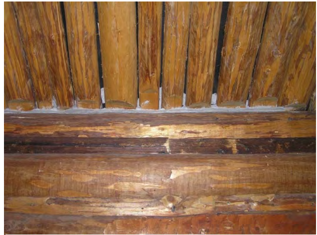
Figure 41: Chinking across the top of the Sleeping Area wall.
