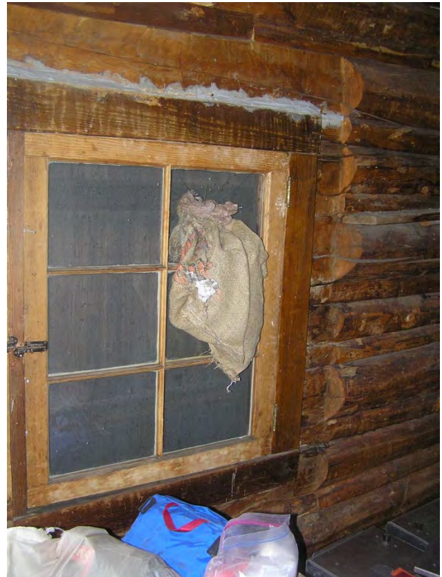
Figure 48: The logs have been beveled and planed to provide a straight substrate for the window trim.
