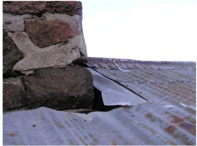
Figure 20: The sheet metal chimney flashing no longer engages the chimney.
