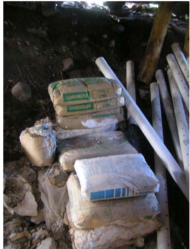
Figure 3: Construction materials left over from the 1993-1994 preservation project, stored in the crawlspace under the Living Area.
