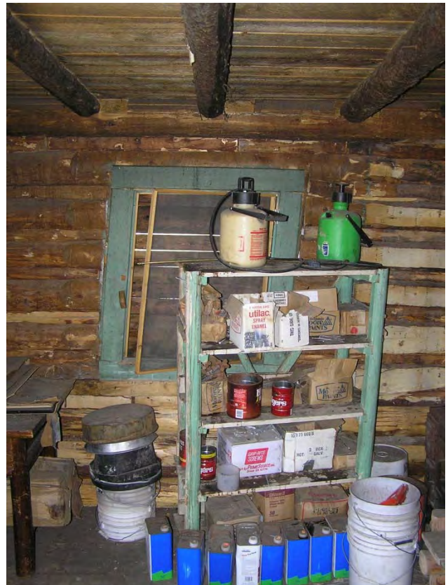
Figure 39: The lower level Kitchen ceiling is the bottom of the exposed flooring above.
