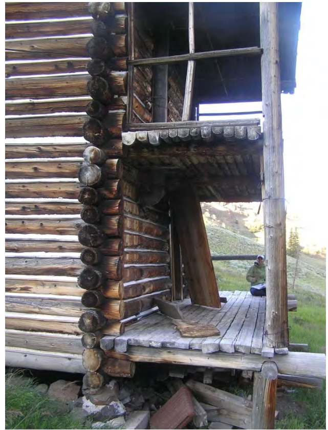
Figure 31: The lower level South Porch, as seen from the west.
