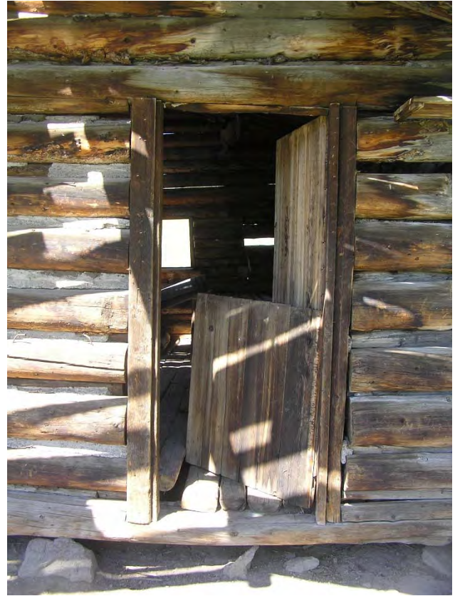
Figure 72: The Dutch door at the north entry into the Cabin.
