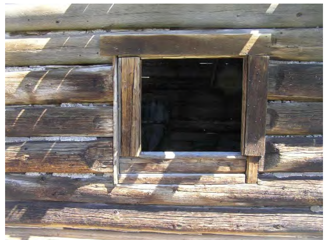
Figure 70: The south window opening was reduced in width sometime after the original construction.
