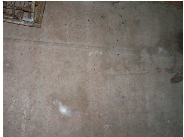
Figure 55: The wood flooring boards telegraph through the sheet linoleum in the Sleeping Area.
