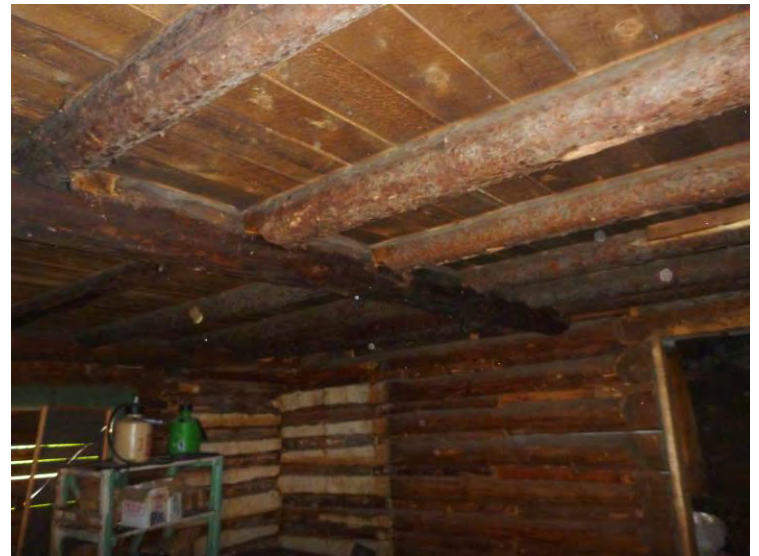
Figure 3: Upper floor framing as seen from the kitchen looking northeast.
