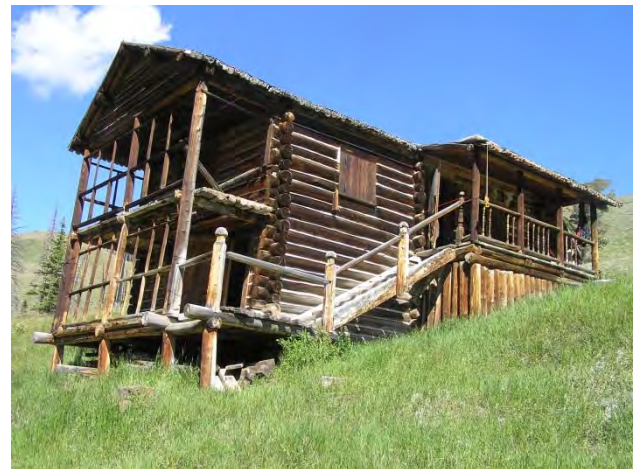
Figure 32: The exterior stairway connecting the main level east porch to lower level South Porch was constructed in 1993-1994.
