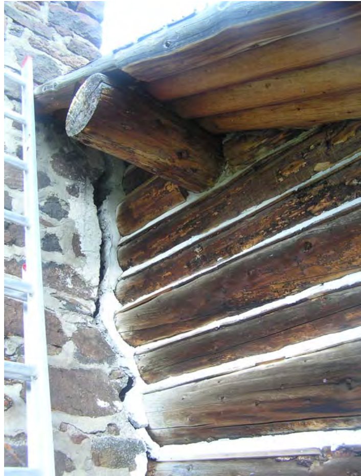
Figure 11: Gap at stone chimney and north log wall.
