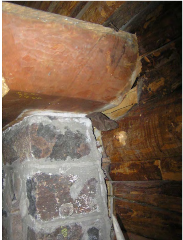
Figure 44: The stone surround of the fireplace has separated from the log wall.
