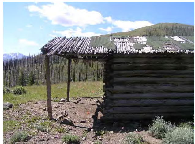
Figure 61: The north slope of the gable roof provides a more complete example of the green membrane roofing that once covered the log poles.
