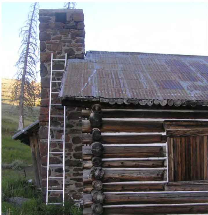
Figure 12: Stone chimney as seen looking east.
