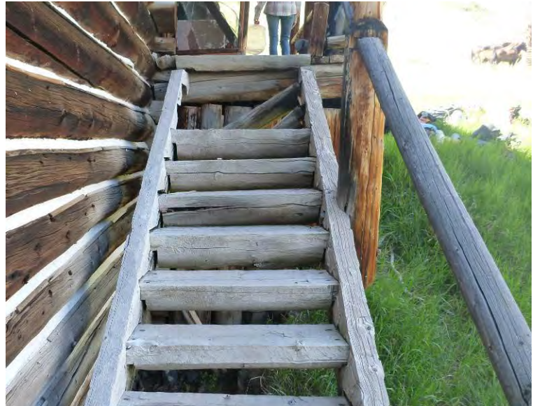
Figure 9: The 1991 stair is exposed to the elements. Logs are deteriorated and spiked connections have failed.
