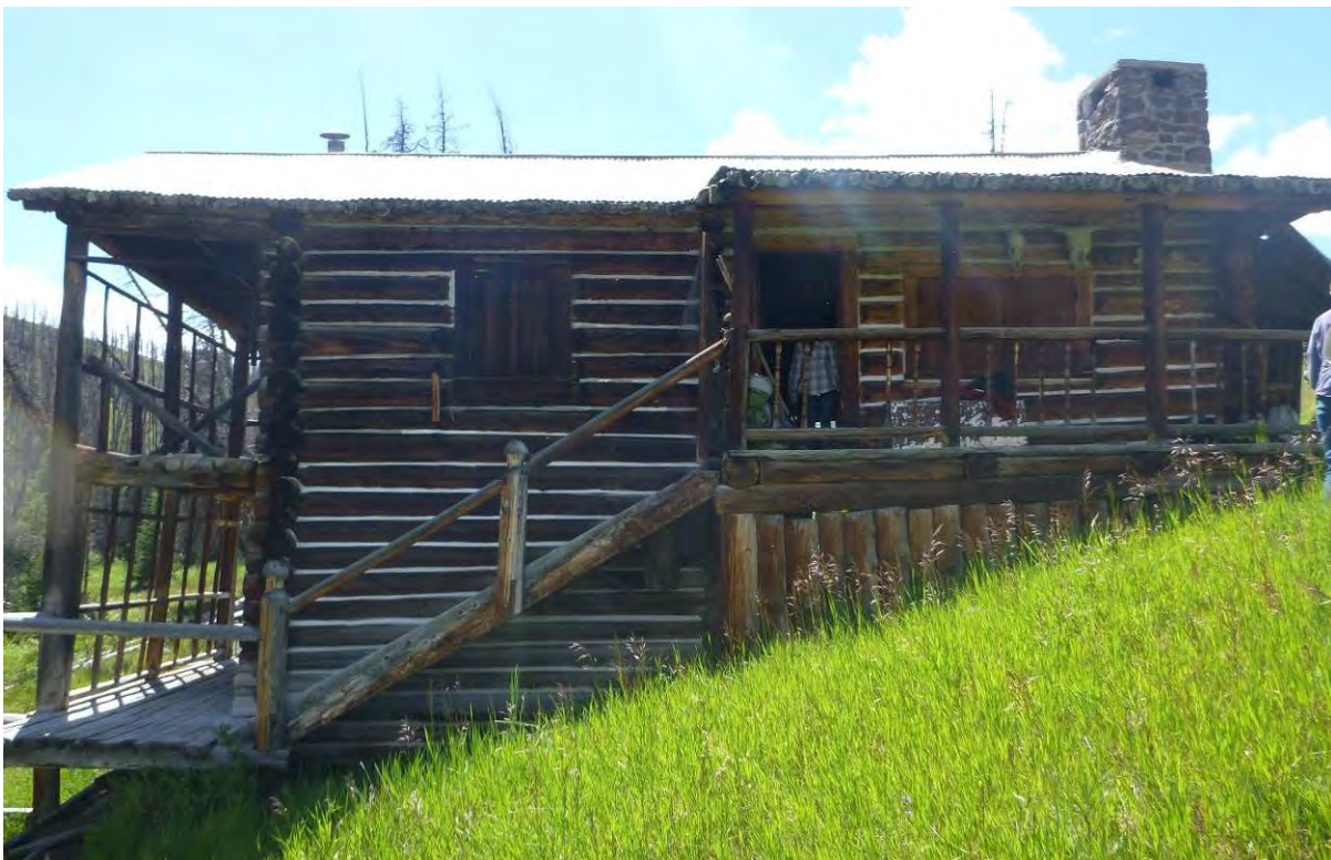
Figure 1: Anderson Lodge east elevation.
