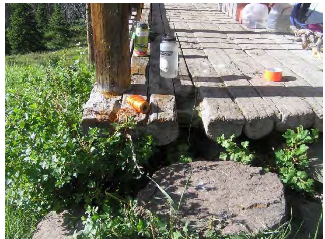
Figure 28: A 1'-4" long portion of the puncheon flooring is missing at the north end of the east porch.
