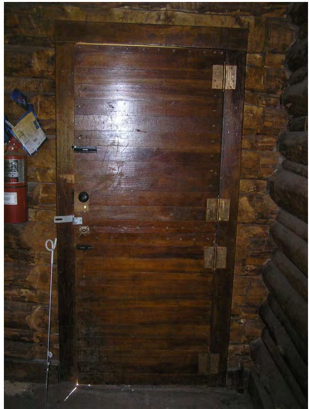
Figure 50: The interior face of the entry door to the Living Area shows the sheen used in the finish on the horizontal boards of both leaves of the Dutch door.
