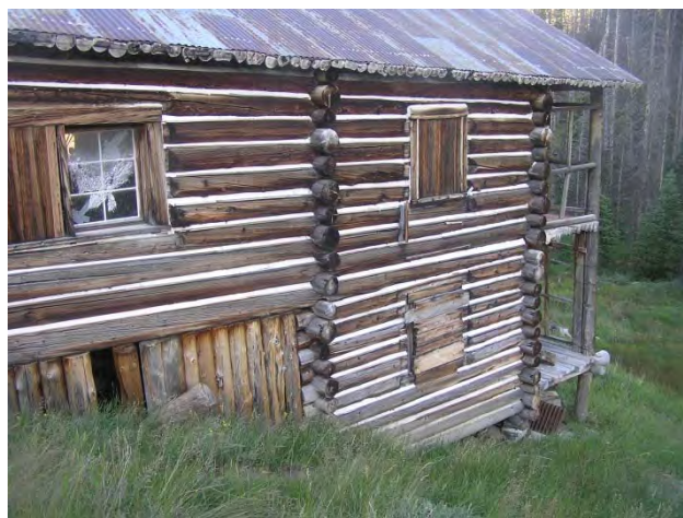
Figure 25: The stockade walls are being pulled down-slope with eroding soil.
