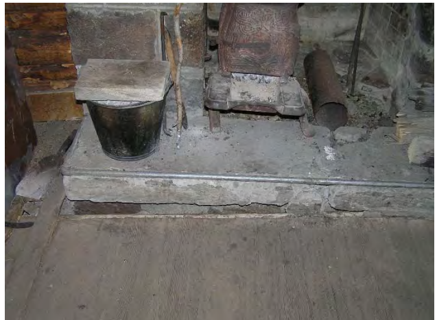
Figure 45: The wood flooring has settled and disengaged from the concrete hearth.
