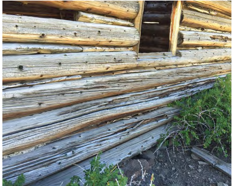
Figure 14: The wall logs at the west elevation are deteriorated and should be replaced.
