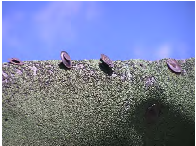
Figure 63: The roofing membrane was fastened to the rake poles with roofing nails and tin caps.
