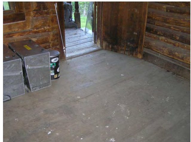
Figure 52: The main level rooms have a simple wood baseboard, as seen on the south wall of the Living Area (looking southeast towards the entry door).
