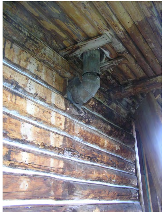
Figure 23: The daubing mortar is missing from the logs at the south wall facing the lower level porch. The wood daubing strips remain.
