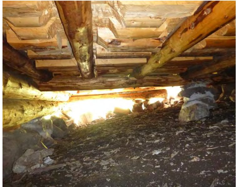
Figure 4: Kitchen floor framing, looking west from the transition to the south porch.
