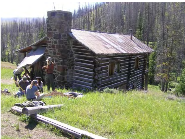
Figure 12: Image of current roofing. Photograph taken from the northwest.
