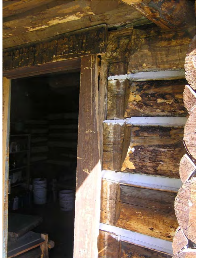
Figure 37: The jamb trim at the entry door to the lower level Kitchen has splintered off.
